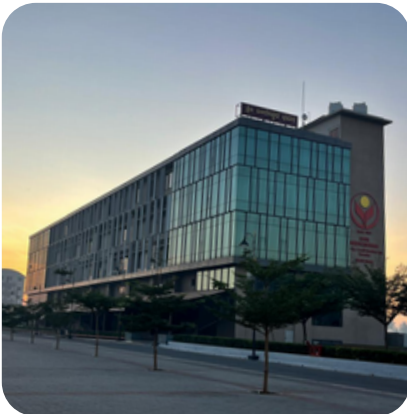
Beereshwar Exam Facility – Ventilation and cooling systems for institutional setup.
