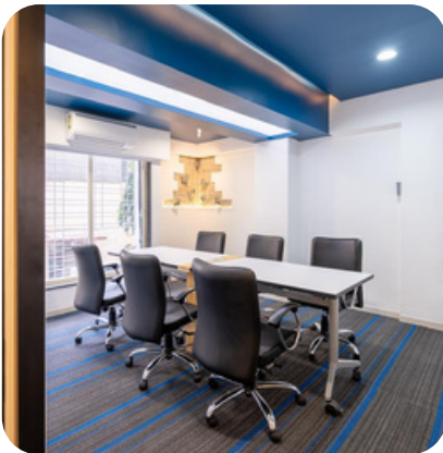
CA Office – Complete HVAC solution for a modern corporate office.
